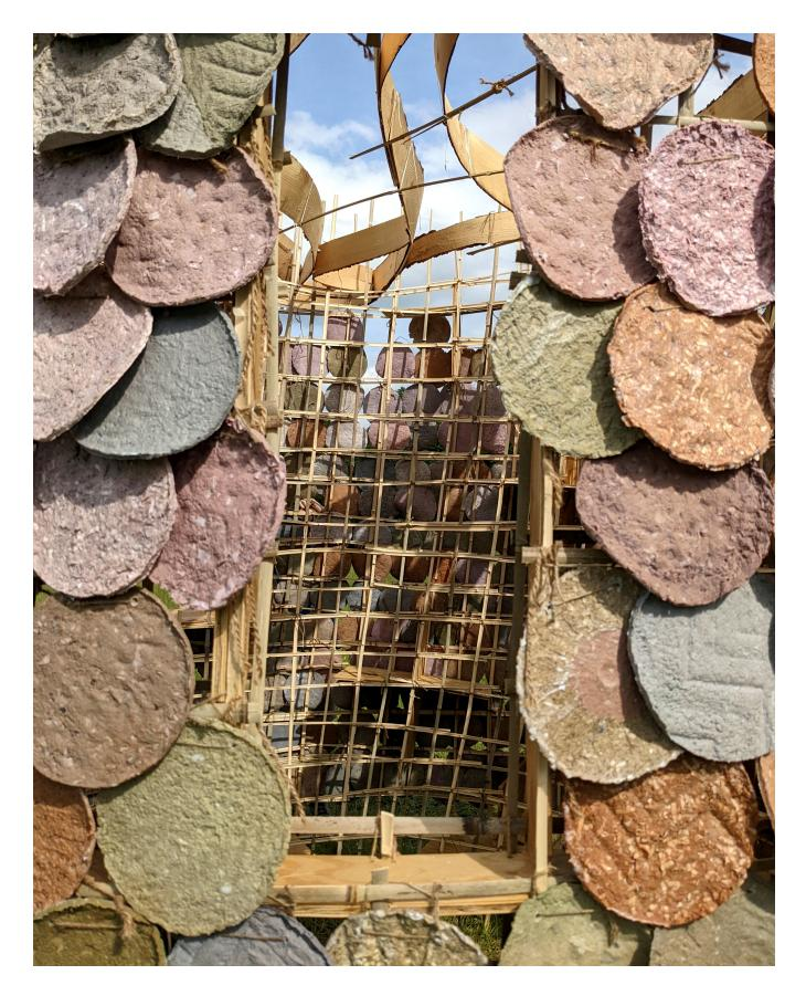
Figure 5. Paper pulp shingle and window detail, with woven bamboo wall visible on the interior.
